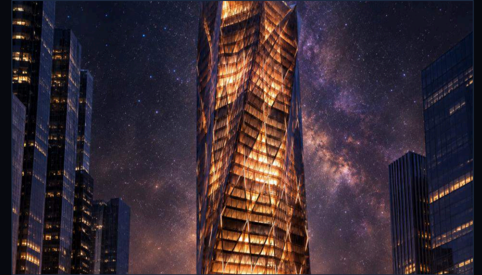
03 VAKIFBANK HQ State bank headquarters · Istanbul, Türkiye
